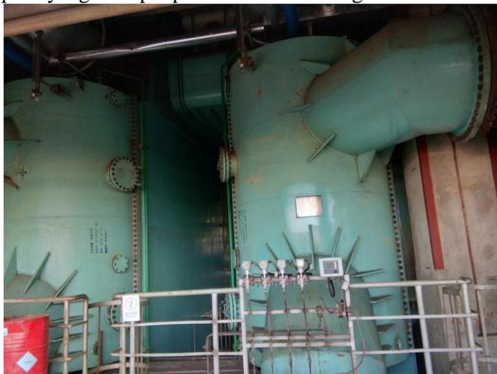
Gambar 1. Kondensor *Surface* Unit 4
