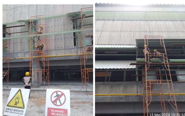
Gambar 4. Scaffolding single pipe
