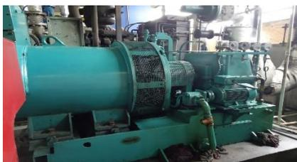
Gambar 1. Turbin Uap – Generator
