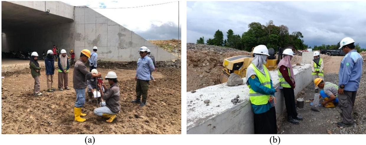
Gambar 3. Pelaksanaan *Quality Control* Pekerjaan Timbunan (a) *DCP Test* ; (b) *Sand Cone Test*
